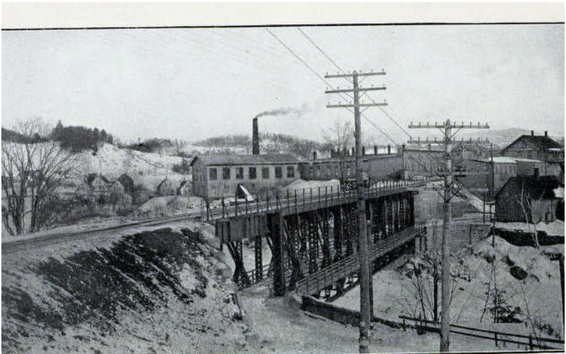
New Steel Bridge, Opened February 1, 1904.
