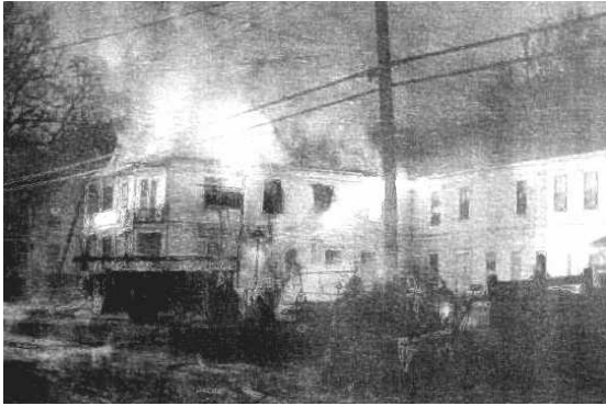
White's Store suffered fire damage in the early 1980's, especially to the living quarters over the store.
