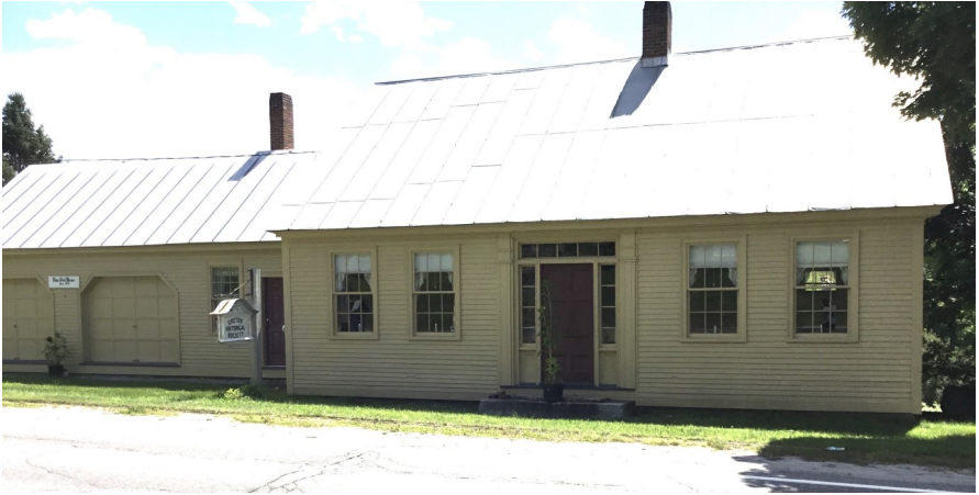
Peter Paul House repaired and painted sans shrubbery. Photo by Lise Shallberg
