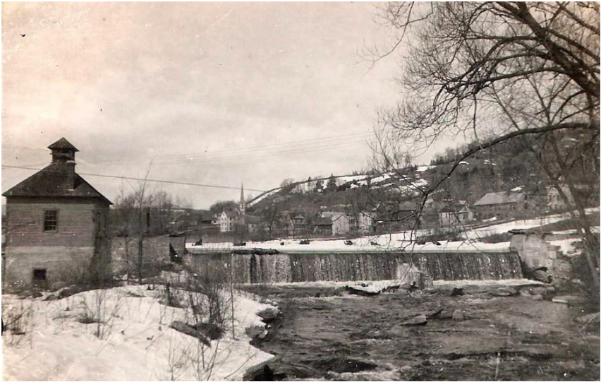
Hydro Electric Generating Plant behind Baptist Church
